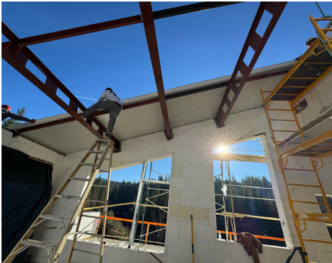
The PHNX Longspan™ Roof and Floor system features beams spanning up to 32 feet, with 8-foot spacing.
